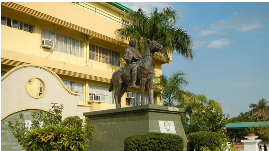
Figure 2: Photograph of WUP Administration Building
